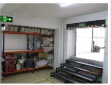
NC photo 2: The height of the 2 emergency escape routes between the washing section and the knitting section of the company is less than 200 cm (with a low ceiling). There are also shuttered doors on 2 emergency escape routes.
