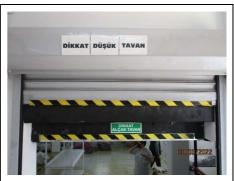
NC photo 3: The height of the 2 emergency escape routes between the washing section and the knitting section of the company is less than 200 cm (with a low ceiling). There are also shuttered doors on 2 emergency escape routes.
